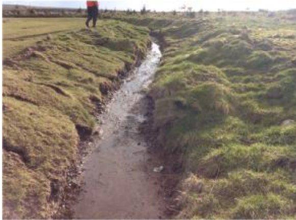
Figure 9: The new ditch to right of 17 has been an excellent introduction and should help improve drainage as well as providing a good outlet for future drainage.
